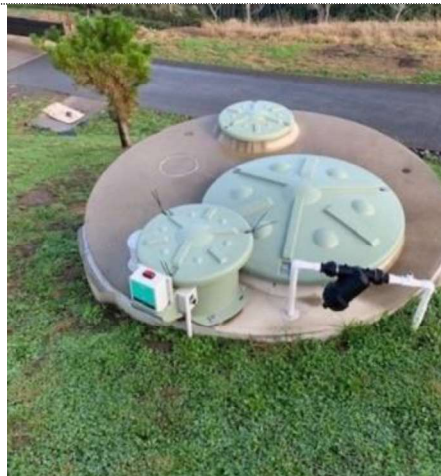
Inspect the tank and surrounding landscape.
